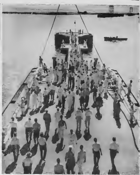
GUESTS INSPECT the new No. 2 Finger Pier as all the ships in the harbor blast a marine salute with their whistles.
